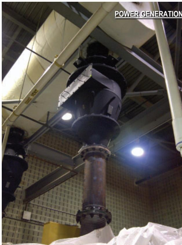
Independent emissions tests required by the Philadelphia Air Management Services showed that the Modulex B80 converters achieved CO reductions that exceeded the minimum 93% limit, the company said.
