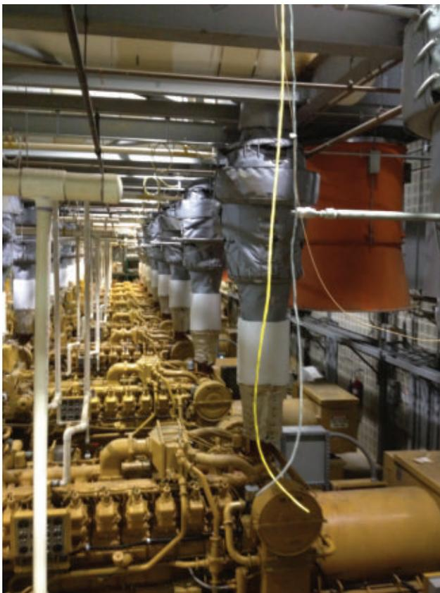
Johnson Matthey said that along with the physical constraints, the pressure drop across the catalytic converter had to be small because the allowable backpressure on the engine was relatively low.
