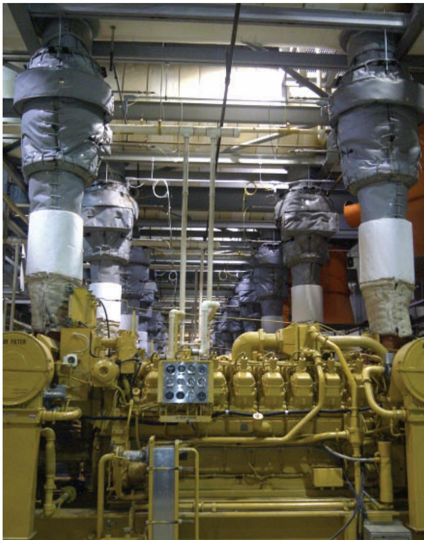
Johnson Matthey's Modulex B80 CO catalytic converters were chosen to help Temple University achieve RICE NESHAP compliance with its 10 sets of tandem Caterpillar 3516 natural gas engines. The limited space in the university's facility made it a challenge to find the right emissions solution, the company said.
